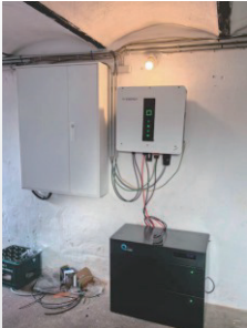
Baden, Germany 12.47 kW PV installed capacity 10 kW hybrid inverter + 10 kWh battery
