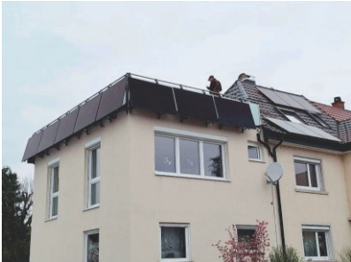
Baden, Germany 12.47 kW PV installed capacity 10 kW hybrid inverter + 10 kWh battery
