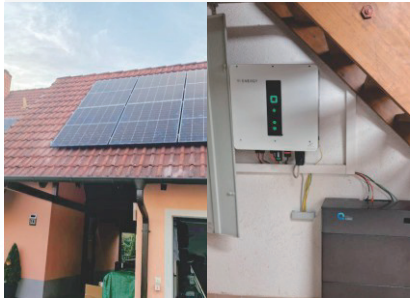
Bamberg, Germany 6.8 kW PV installed capacity 5 kW hybrid inverter + 10 kWh battery
