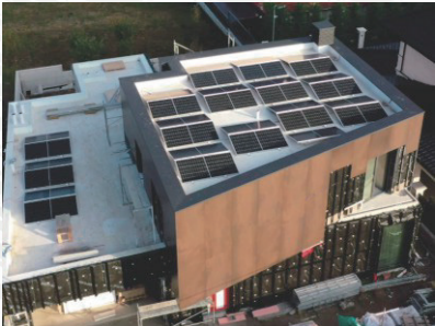
Kishinev, Moldova 10 kW PV installed capacity 8 kW hybrid inverter + 10 kWh battery
