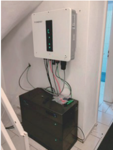
Düsseldorf, Germany 6.66 kW PV installed capacity 5 kW hybrid inverter + 10 kWh battery
