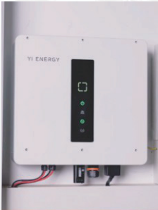
Kishinev, Moldova 10 kW PV installed capacity 8 kW hybrid inverter + 10 kWh battery
