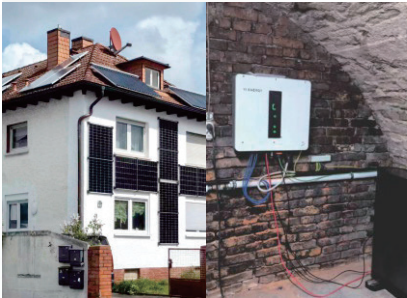
Wiesbaden, Germany 6.64 kW PV installed capacity 5 kW hybrid inverter + 10 kWh battery
